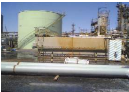
Basin in petrochemical complex
