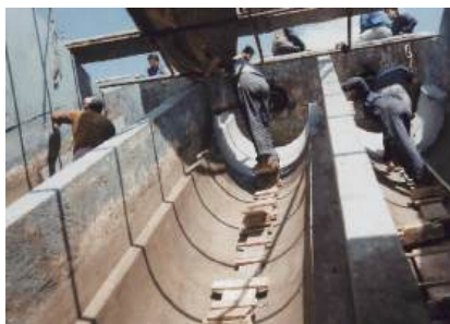
ARC 791 applied to properly prepared surfaces
